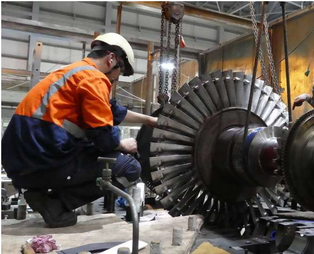
TBFP Rotor installation
