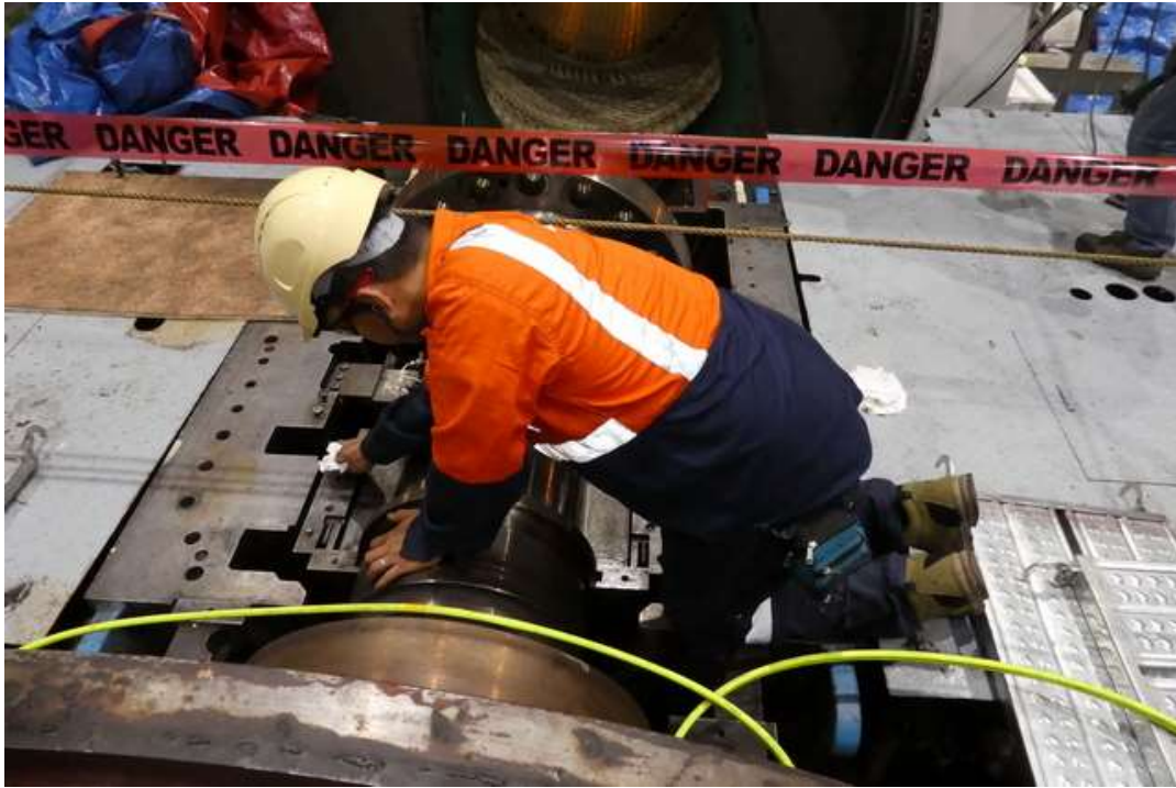
No4 Bearing Reassembly inspection
