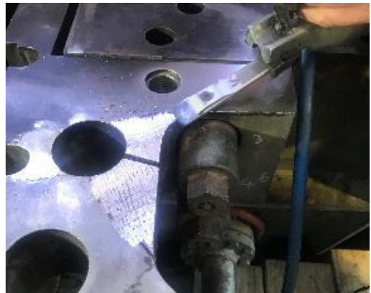
Figure 6 Scraping of the casing to improve clamping
